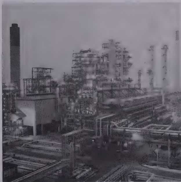
Part of the Shell oil refinery at Ellesmere Port in the UK. The central area of the photograph is dominated by the catalytic cracker plant.
