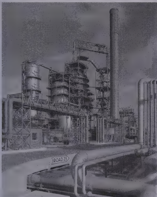
Part of an oil refinery. The fractionating column is on the left.
