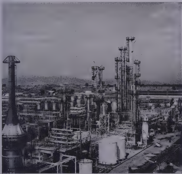
This large chemical plant near Bombay in India can process 225 000 tonnes of naphtha per year. The naphtha is converted into ethene, propanone, PVC, and many other chemicals.
