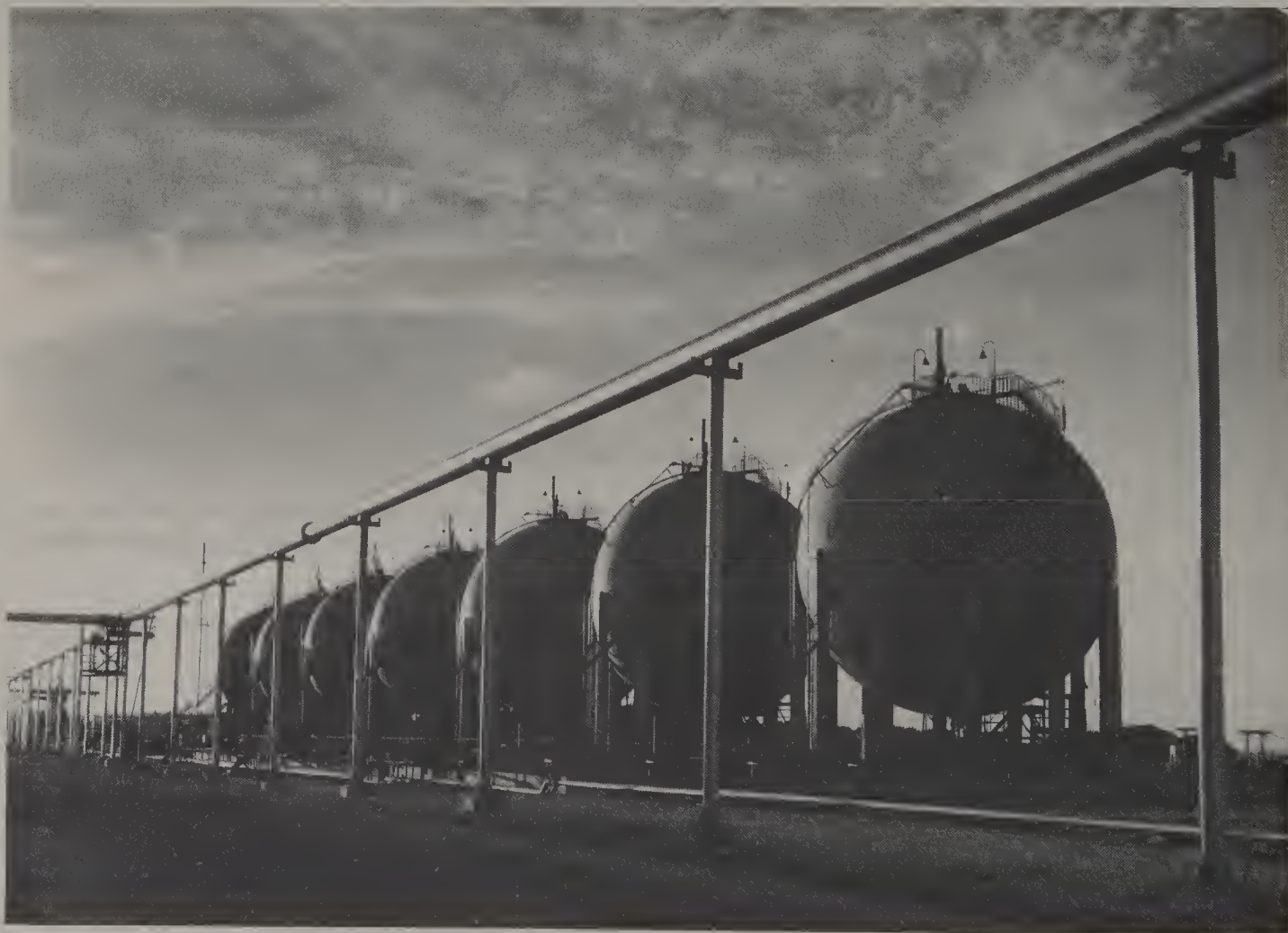
Plate 6.2. Hortonspheres used to store liquefied gases (for example, ethene, propane and butanes, chloroethene) (Esso Petroleum Co. Ltd.)
